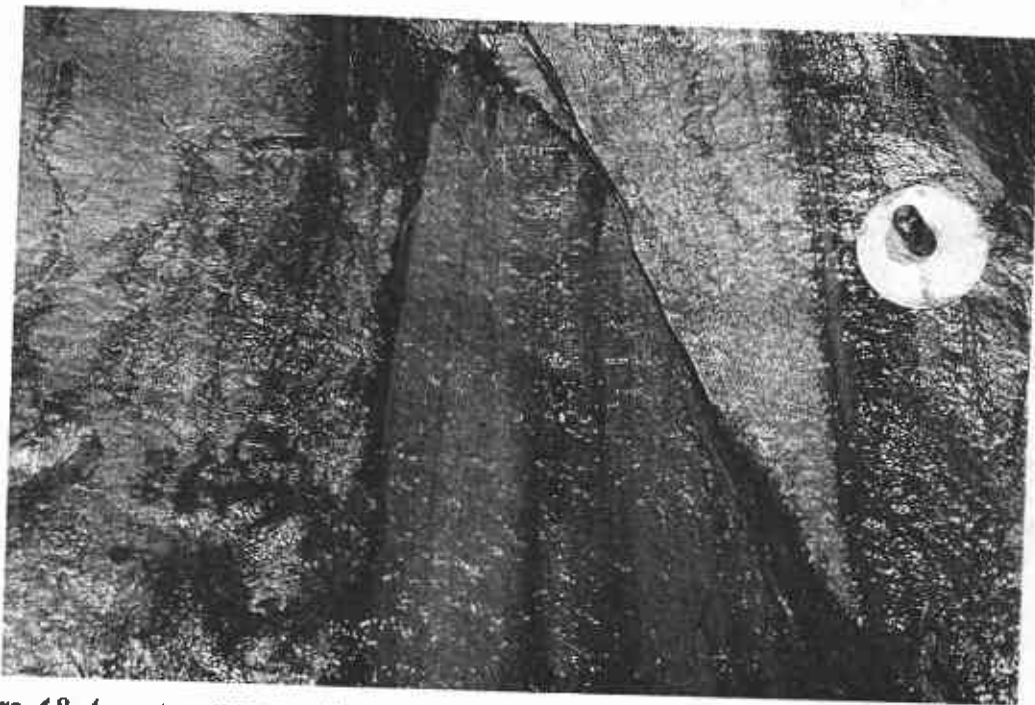
Figure 4.8 A water transporting fracture with a slimy "curtain" of iron oxidizing bacteria. The light brown colour indicates a young precipitate with an active oxidizing population. As such precipitates ages, it turns dark brown and brittle. The precipitates will be dark brown to black if manganese oxidation is ongoing. The picture is from the Åspö tunnel, the A side, length 1993 m. And was taken the 6 of June 1993.
